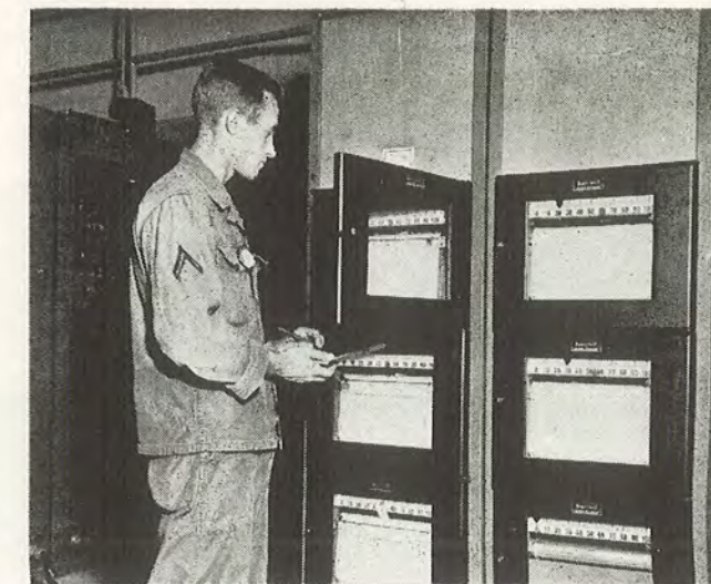
A Signal Corps technician checks the recording instruments where a continuous record of chain operation is plotted, enabling engineers to assess the operation of the system.
